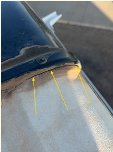
sealant failing
