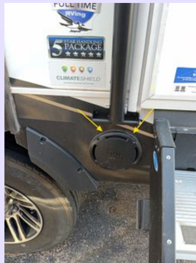
location where sealant is cracked
