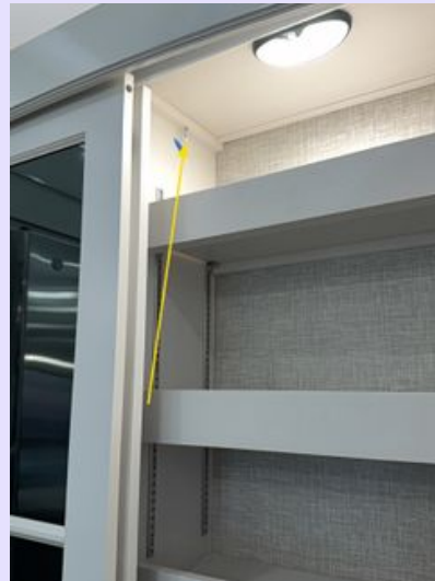
Location of screw backing out
