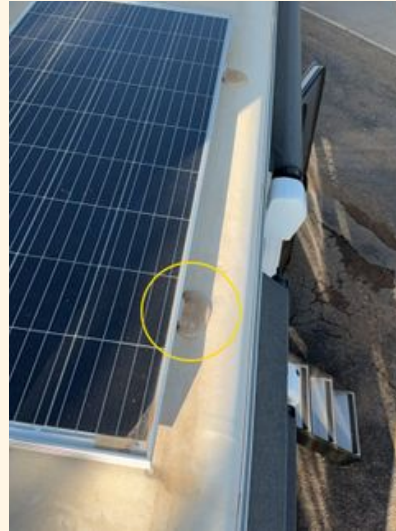
Area where air bubble is present
