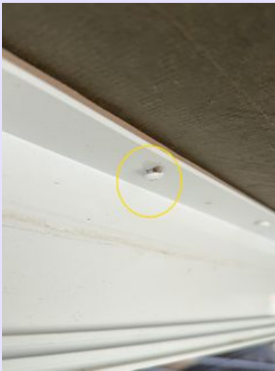
screw poking out, not all the way in.
