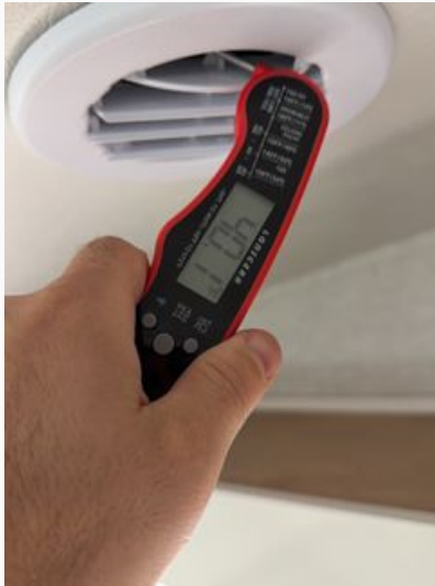
Air discharge temperature 40.1 F
